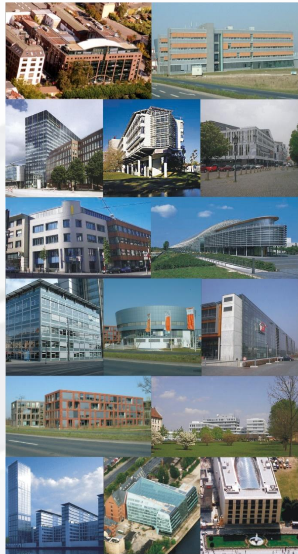
Figure 4: Evaluated SSF buildings in Germany.
